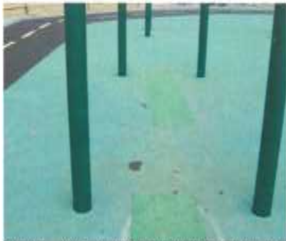
Photo 3 - Material applied adequately to edges of equipment. Note patching of VitriTurf.
