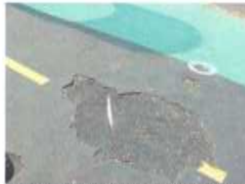
Picture 1 – Typical worn or damaged VitriTurf
