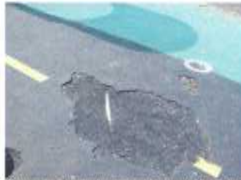
Picture 1 – Typical worn or damaged VitriTurf
