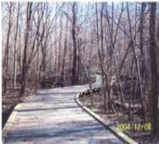
Figure 7 - A boardwalk is a design technique used for minimization of impacts through the woods.
