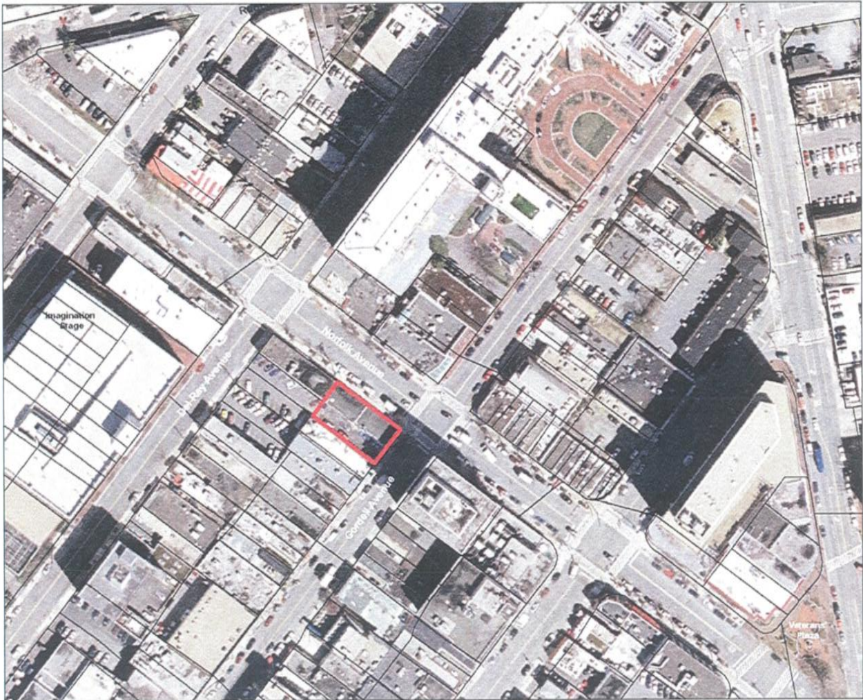
Site Aerial View
