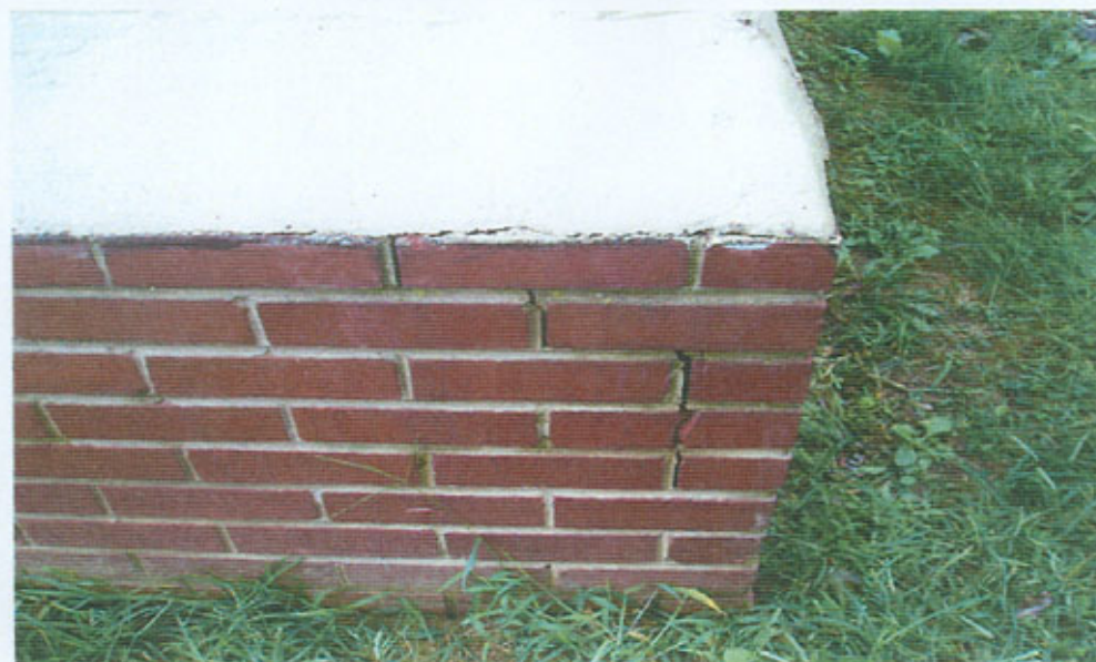
PHOTOGRAPH 3: Minor Cracks in Exterior Brick and Mortar Joints
