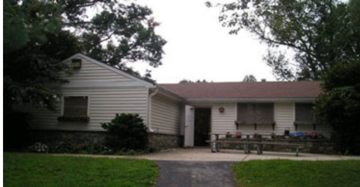
Figure B-1: Westmoreland Hills Recreation Building
