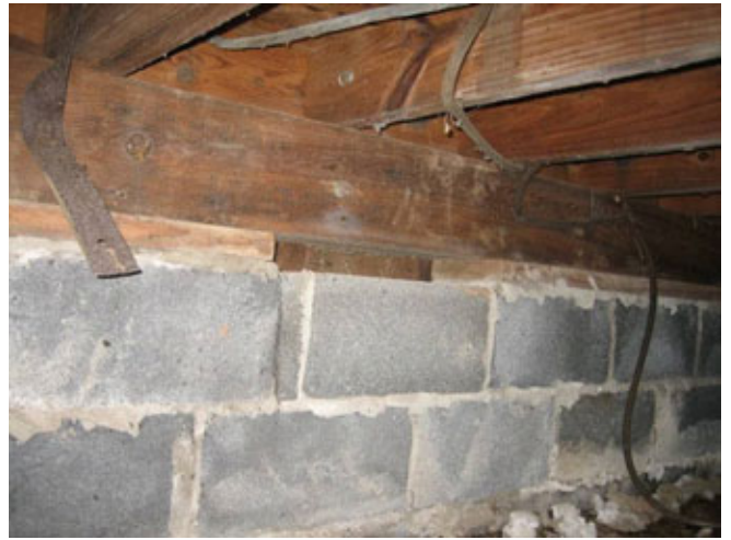
Figure C-7: Crawl space wall
