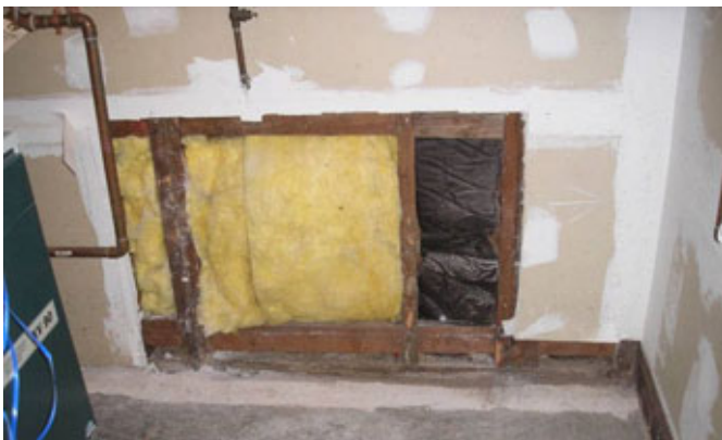
Figure A-7: Mechanical room wall opening
