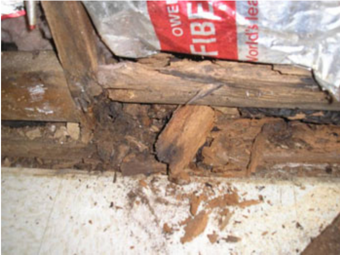
Figure A-6: Significant deterioration
