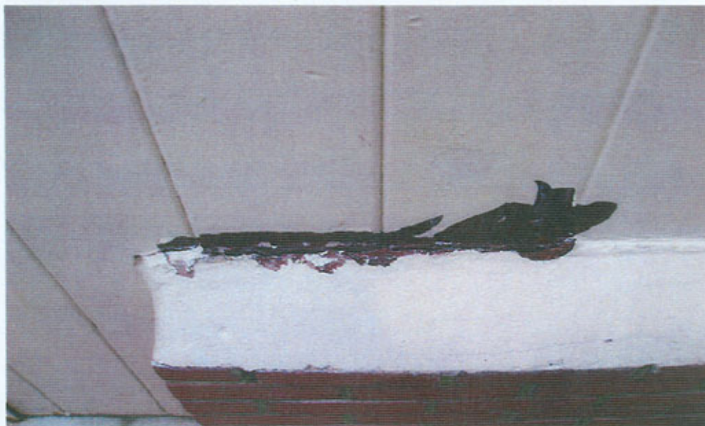
PHOTOGRAPH 2: Area of Expected Exterior Wall Water Infiltration
