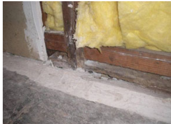
Figure A-8: Mechanical room wall opening
