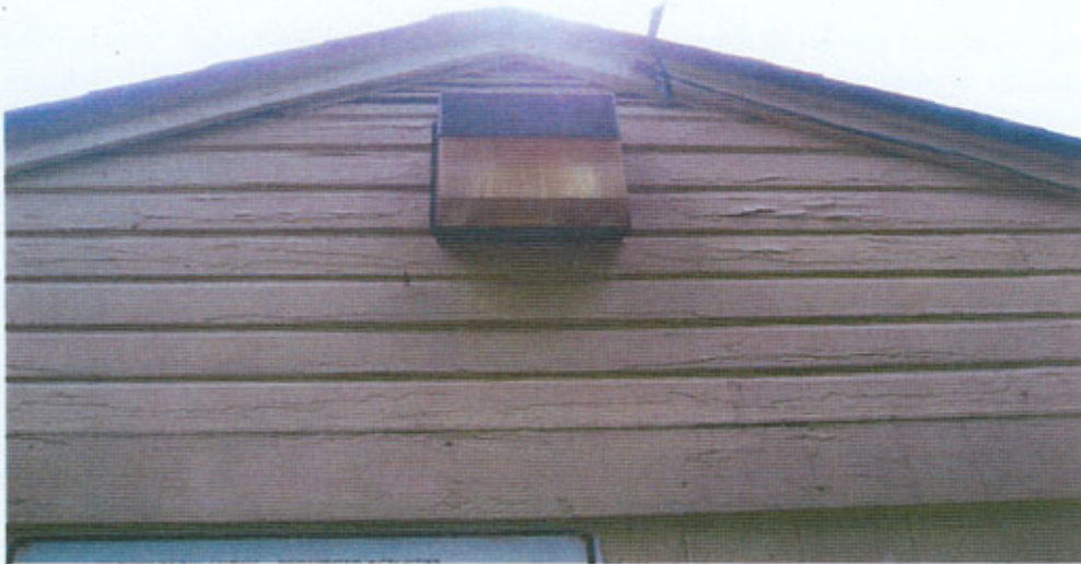
PHOTOGRAPH 1: Exterior Paint Peeling on Gable End Siding
