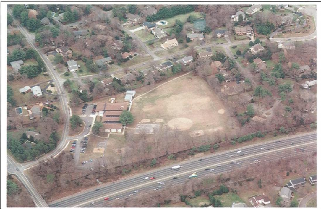
Aerial photograph of the existing Carderock Springs Elementary School, as viewed from the south-southwest. Note the site's forestation that adjoins the Capital Beltway right-of-way on the south.
