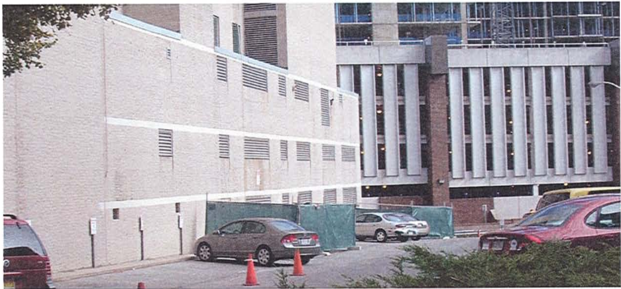
Garage Vents on North Property Boundary
