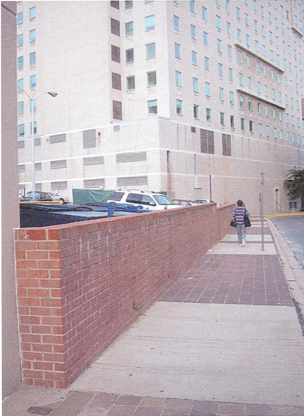
Retaining Wall, from Cameron Street, with Scale Figure
