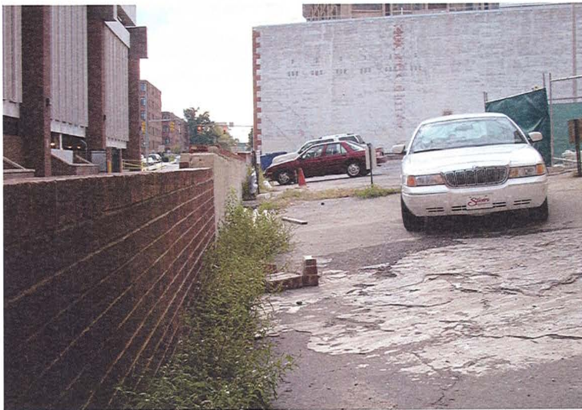
Retaining Wall, from Subject Site
