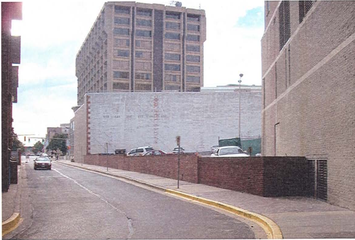
Parking Garage 2 Driveway, with Retaining Wall, looking South
