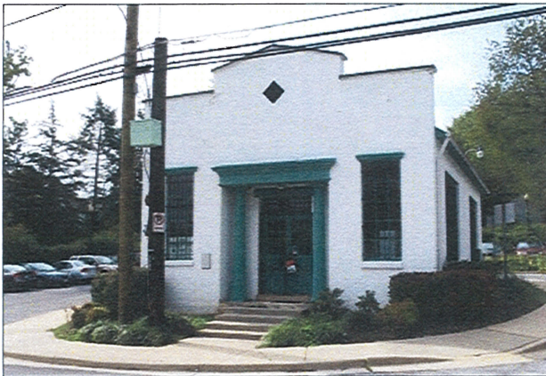
Germantown Bank, 1922, brick structure 19330 Mateny Hill Road
