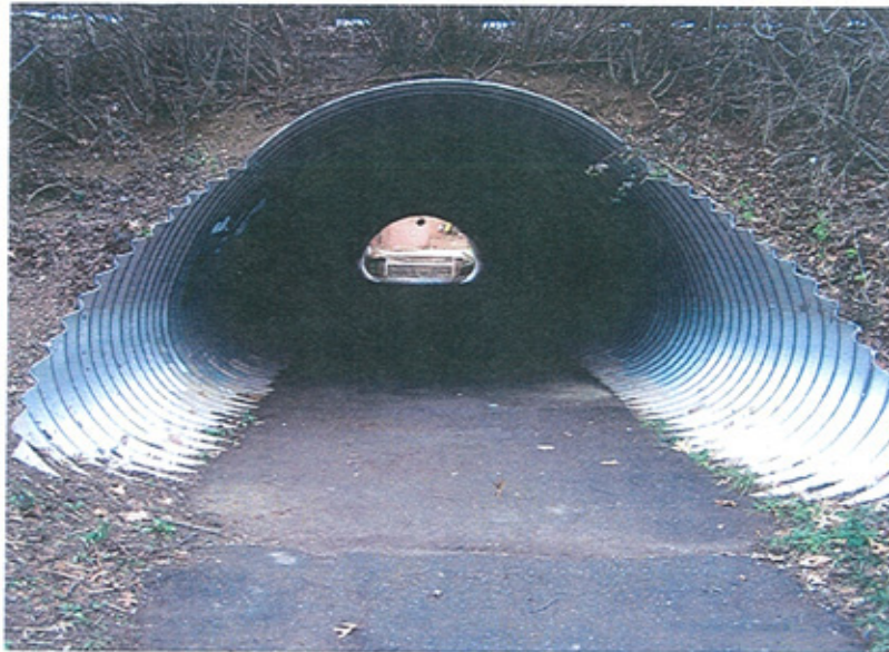
A view looking north through the tunnel before it was barricaded
