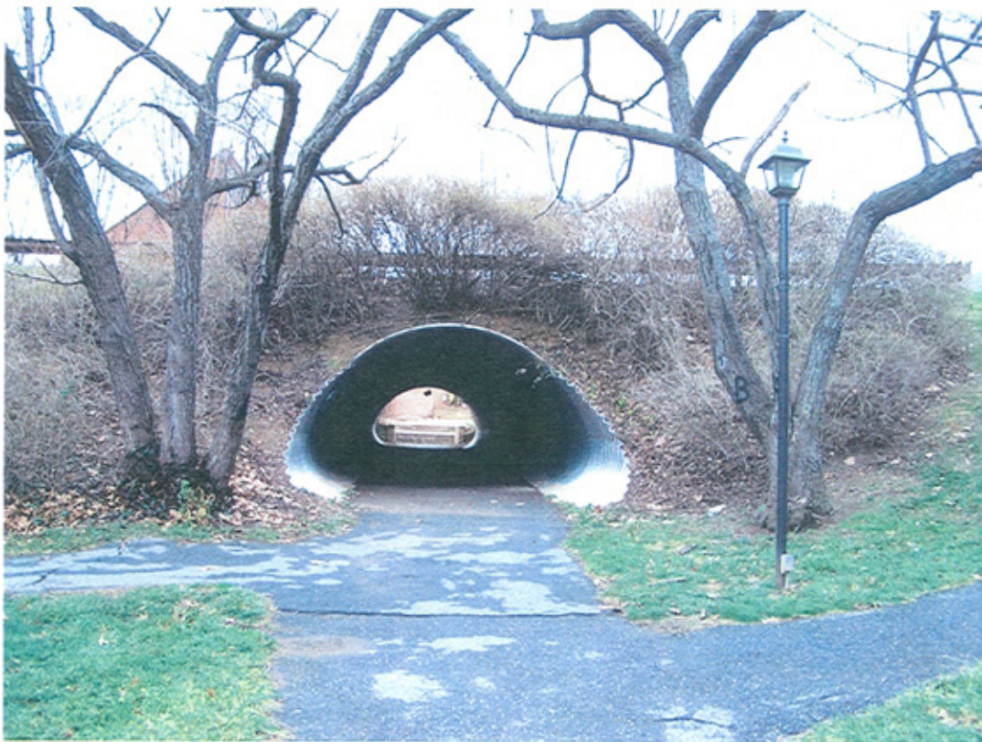
The sidewalks leading into the tunnel on the south sides
