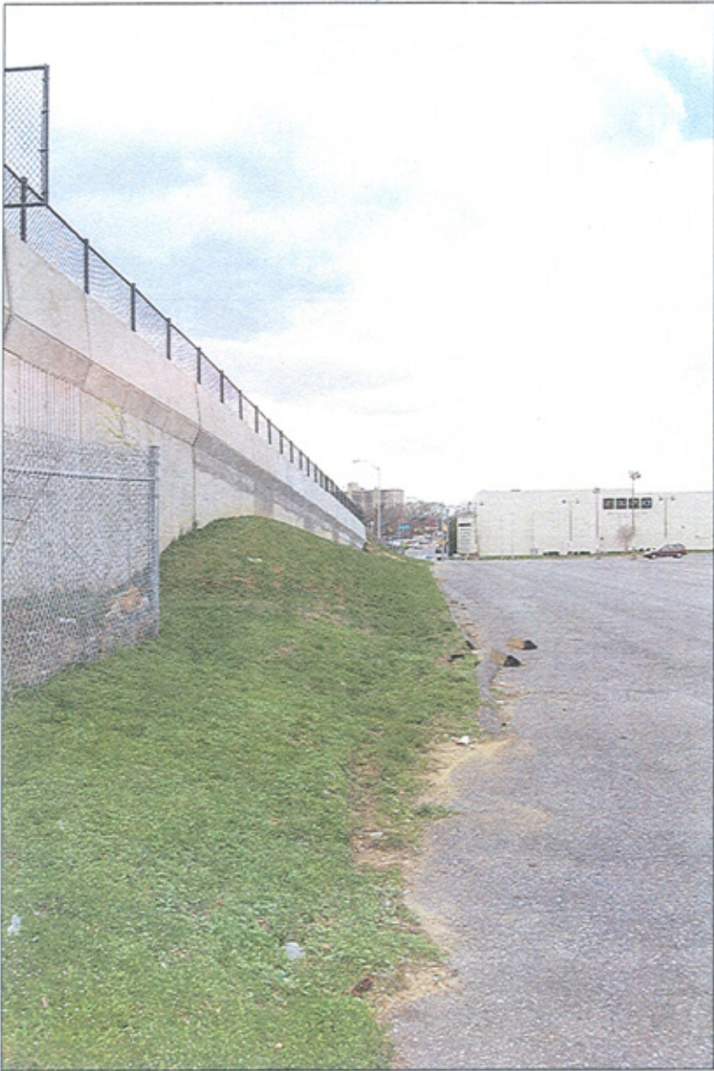
Looking west along the Westlake Terrace overpass
