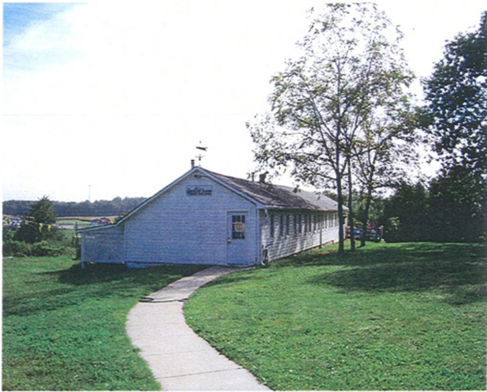
10. Existing "Chicken Coop" used for Trades (facing east)
