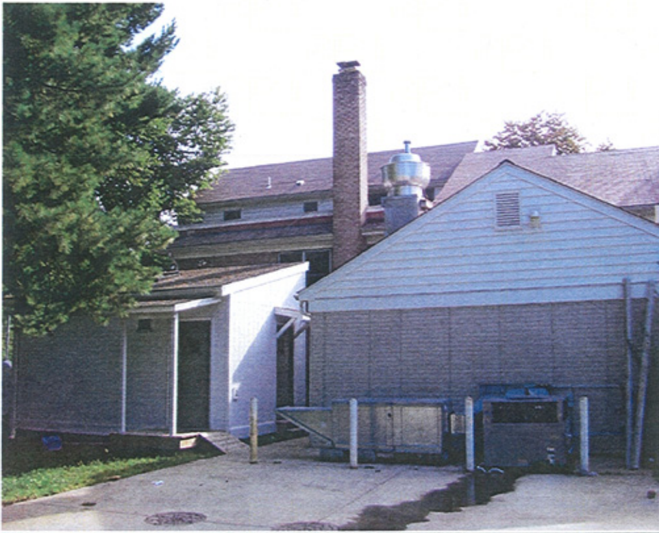
8. Back of existing dormitory (facing east)
