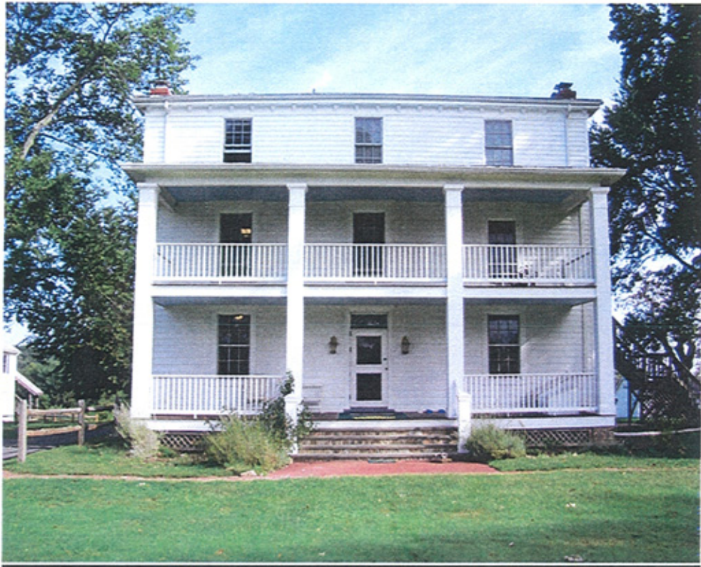
5. Front of existing Farmhouse used for administrative offices (facing north)
