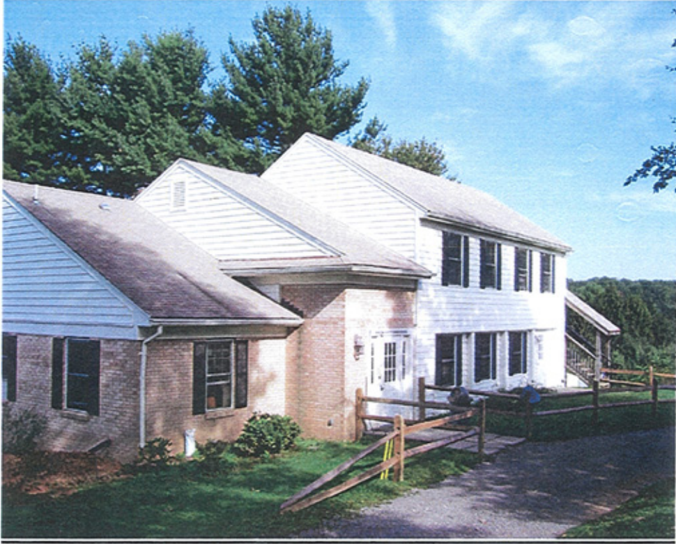
7. Front of existing dormitory (facing northwest)
