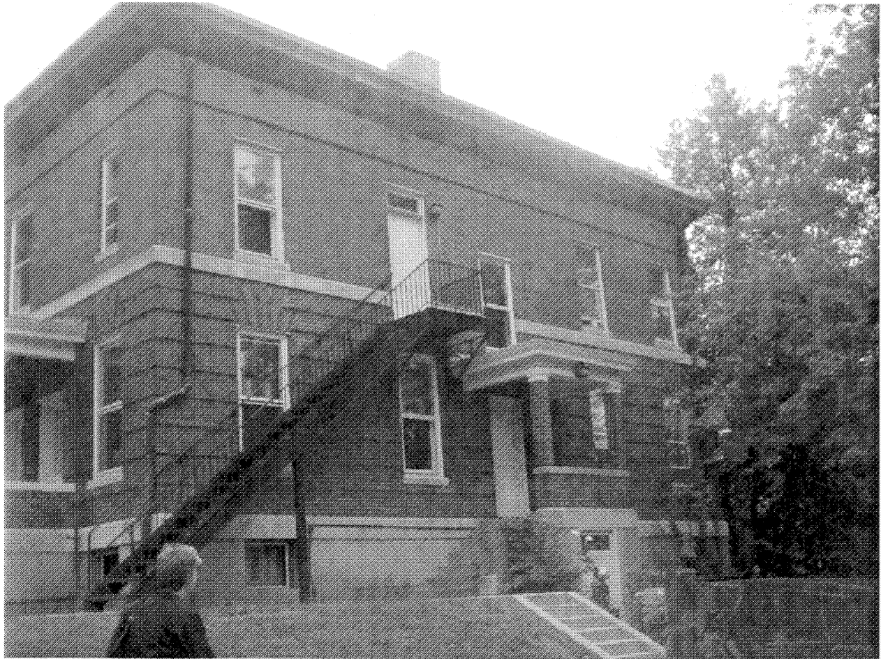
#35-119, Bureau of Animal Industry Building West (Rear) Façade, 10-9-2007
