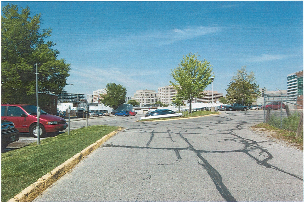
Parking Lot 3, from Fenton Street entrance
