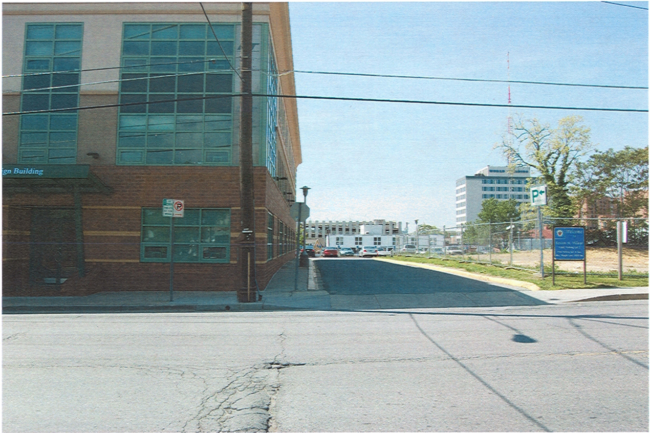
Parking Lot 3 entry from Thayer Avenue, proposed location of new private street
