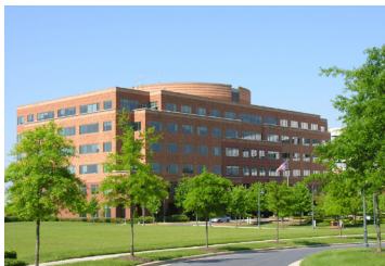
Multi-story office building in the Milestone North Business Park.
