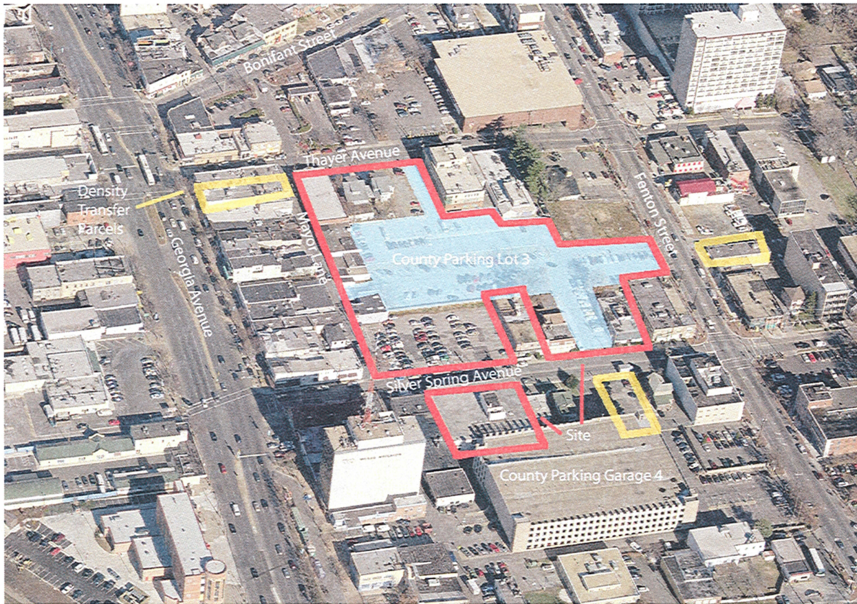
Aerial Photo Looking North
