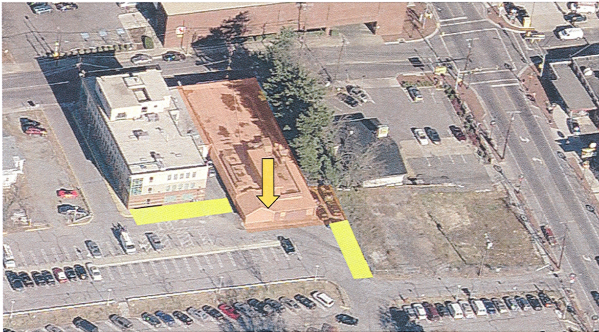
Aerial view of the Kalivas building
