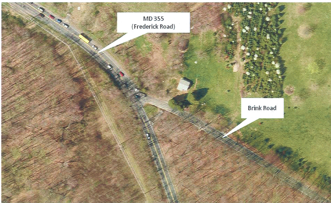
Figure 1: 2008 Aerial Photograph of MD 355 and Brink Road Intersection
