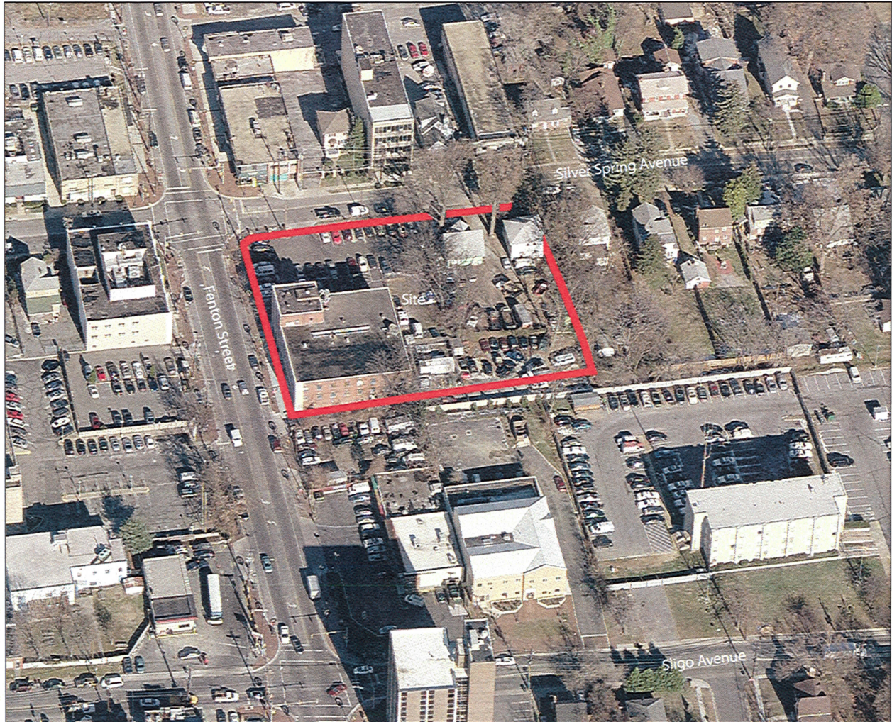
Aerial Photo Looking North
