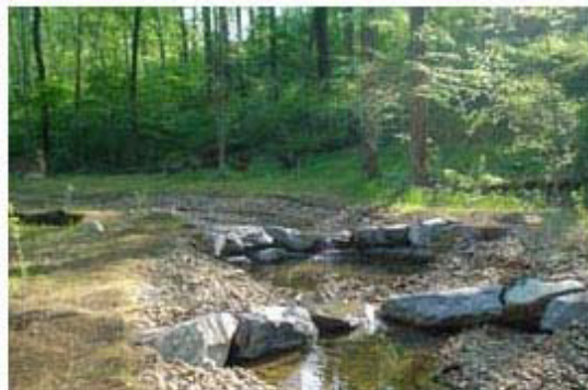
After view showing newly installed step pools
