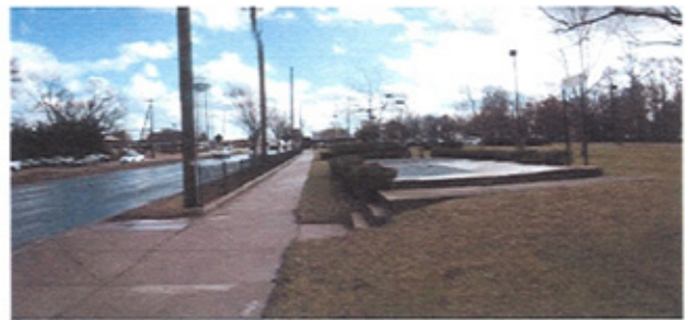
West sidewalk along Georgia Avenue
