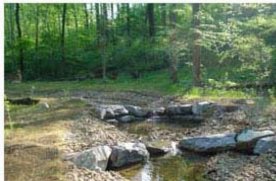
After view showing newly installed step pools
