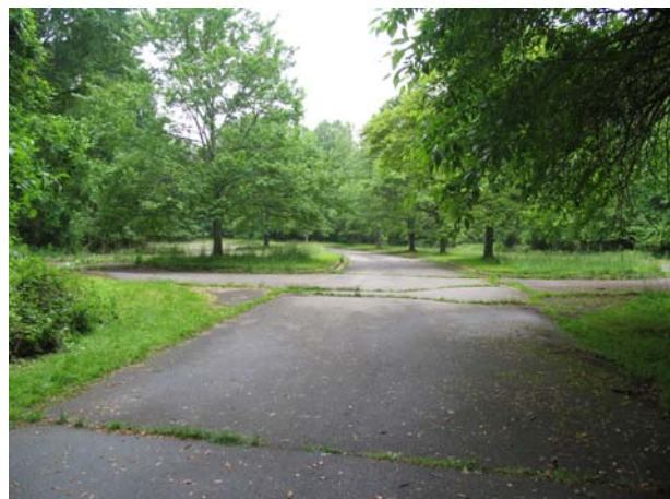
Existing road and parking lot on east side of Lake Frank
