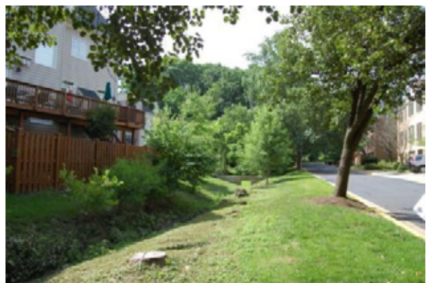
Looking south towards the weir (area “below the weir”)
