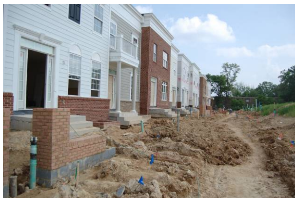
Construction activities onsite
