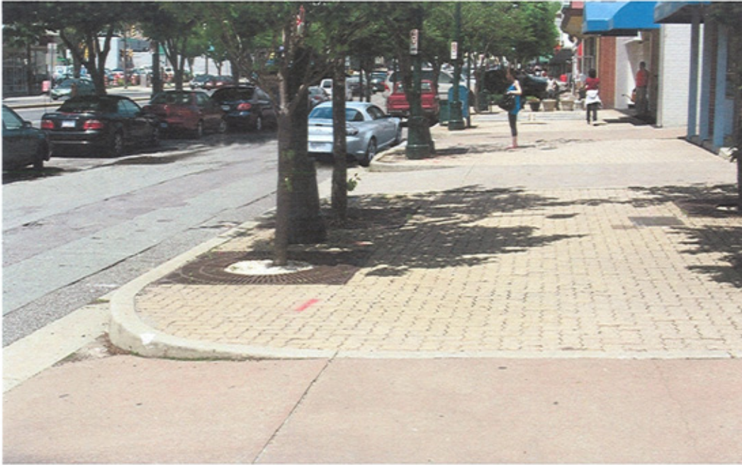
Before View with Concrete Paving and Excessive Cross Slope
