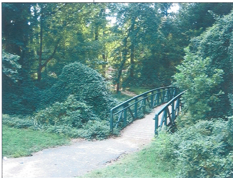
The existing Long Branch Bridge.
