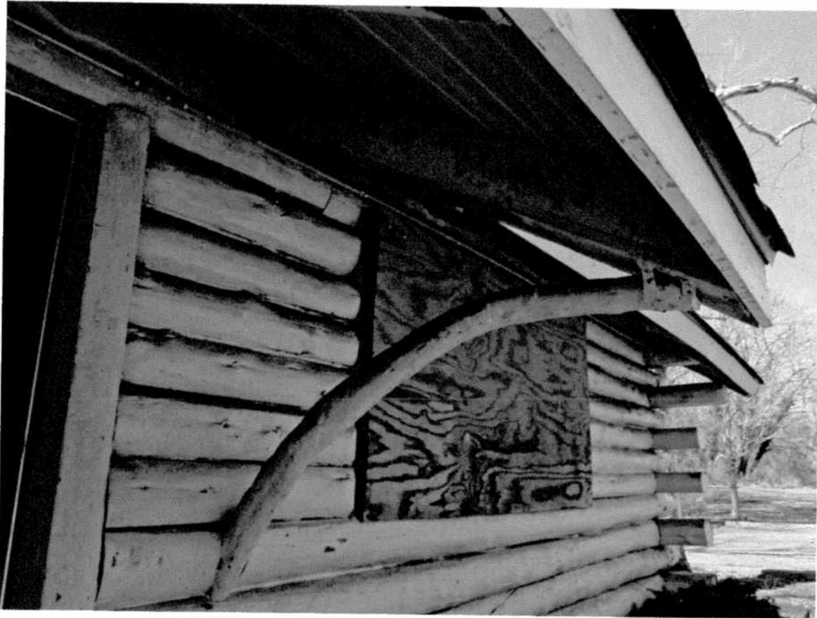
Photo #5: Detail of tree branch brackets at Entry Porch, Kensington Cabin, March 18, 2010 (photograph by Jennifer Gurney, M; 31-41_2010-03-18_05.tif).
