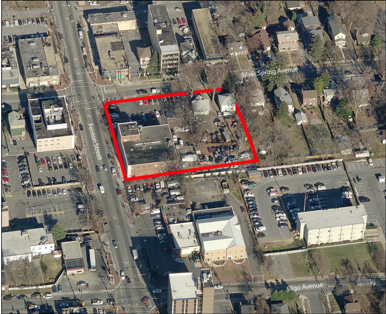
Aerial Photo Looking North
