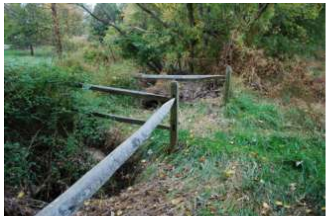
The old culvert and bridge
