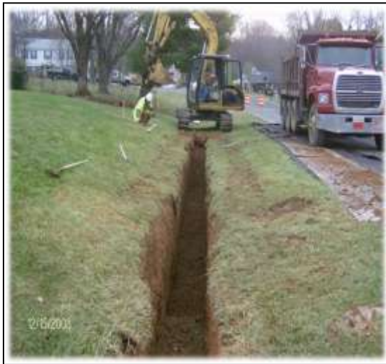
Biotrench in Construction
