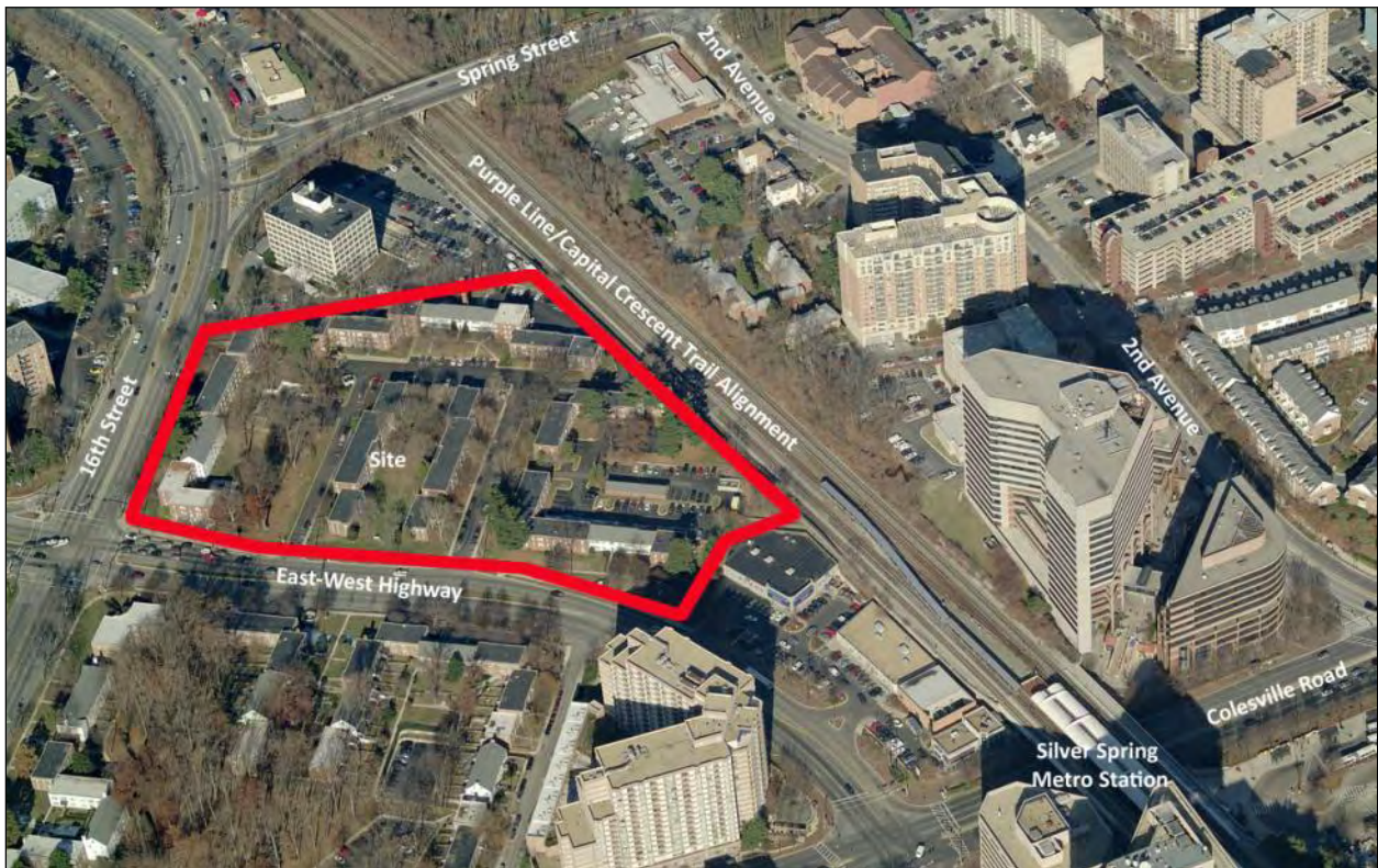
Aerial Photo Looking North
