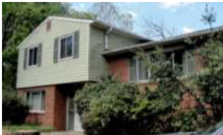
Top - rear view of Riley Farm log wing Middle - front view of Riley Farm Bottom - the Rozier property house
