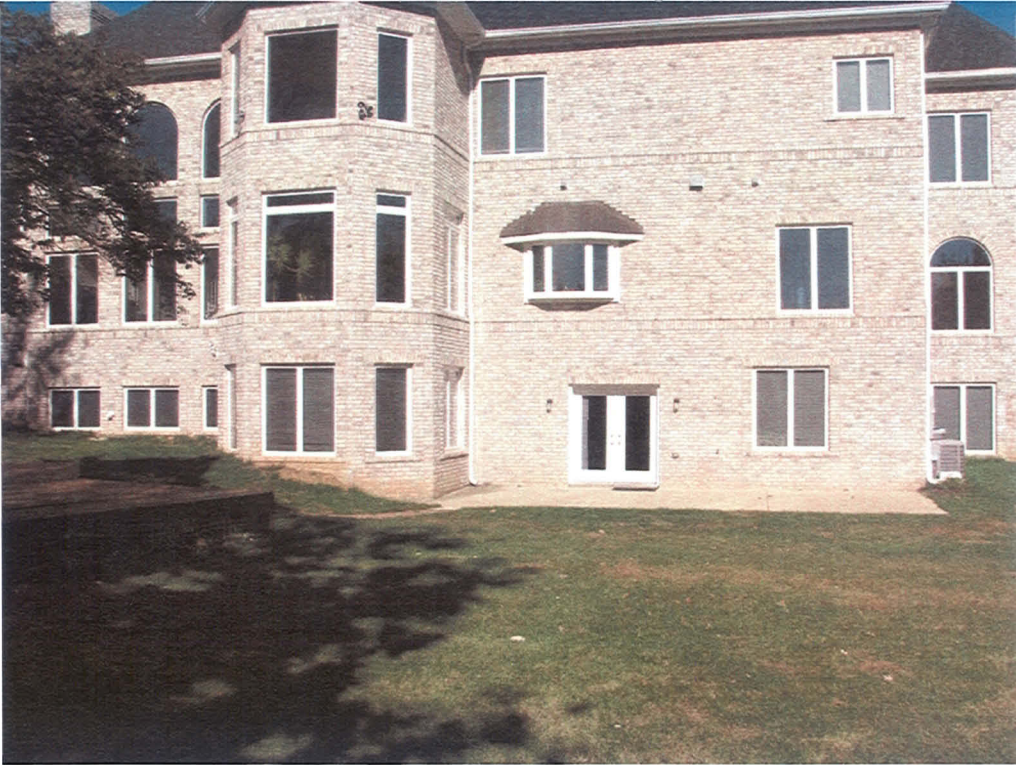
Figure 5: Entrance to Child Care Facility (Rear View of Property)
