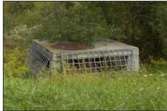
Photo 1. Example of a riser structure.
