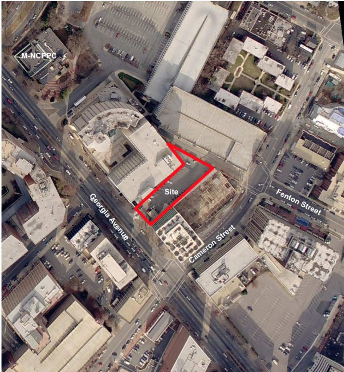
Aerial Site View
