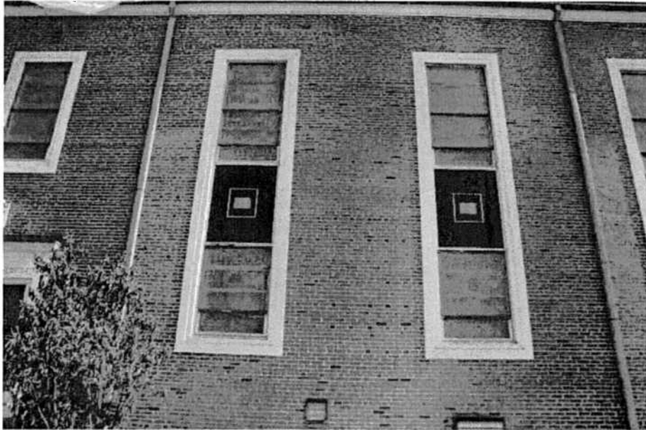
Silver Spring Baptist Church, west (side) façade detail, Clare Lise Kelly, 02.19.10
