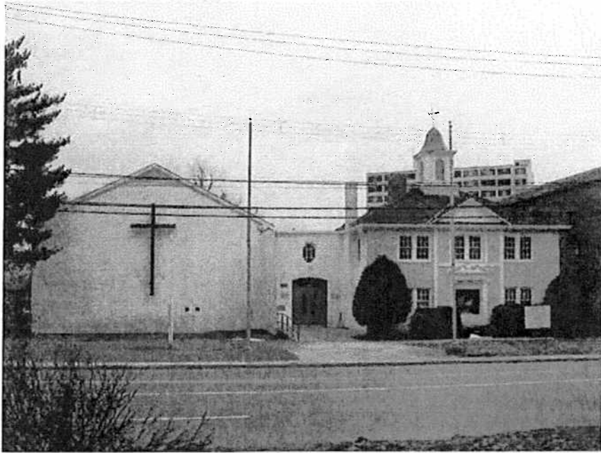
Silver Spring Baptist Church, parsonage and addition, north façade (front), Lisa Mroszczyk, 03.10.10
