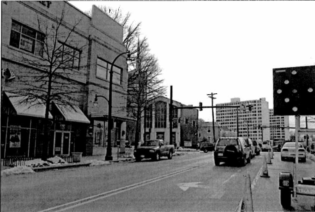
Figure 33. View towards First Baptist Church of Silver Spring from mid-block north on Fenton. February 2011.
