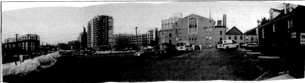
Figure 30. Panoramic view of the church's rear facade and recent encroachment. February 2011.
