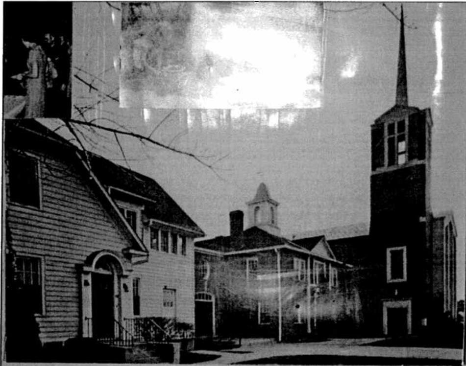
Figure 13. First Baptist Church of Silver Spring. Former education building (left) demolished in 1976.
