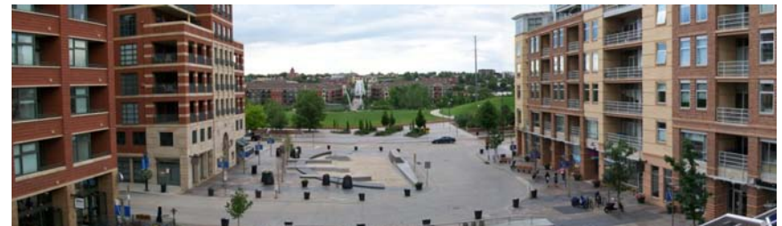
Boundary between two Neighborhoods
