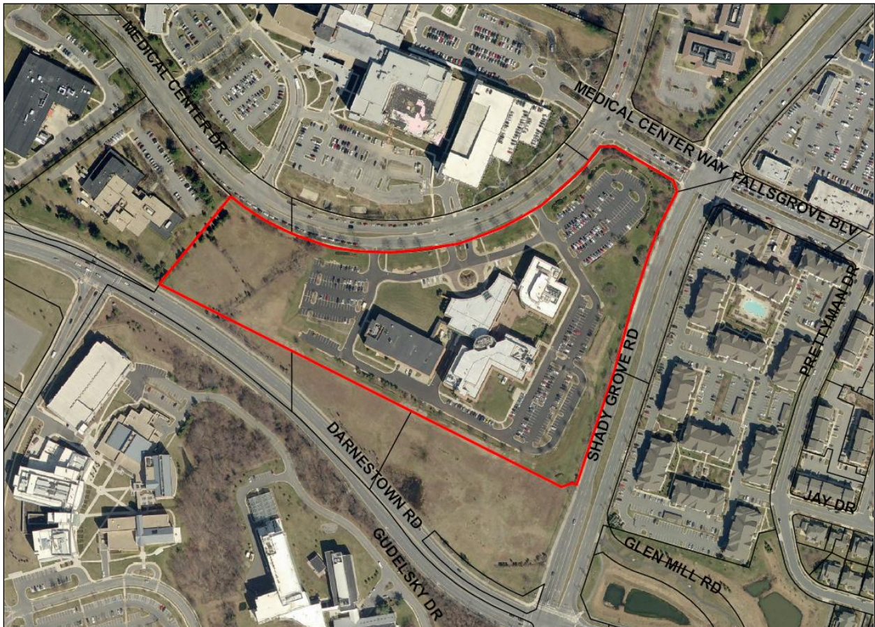
Site Aerial View
