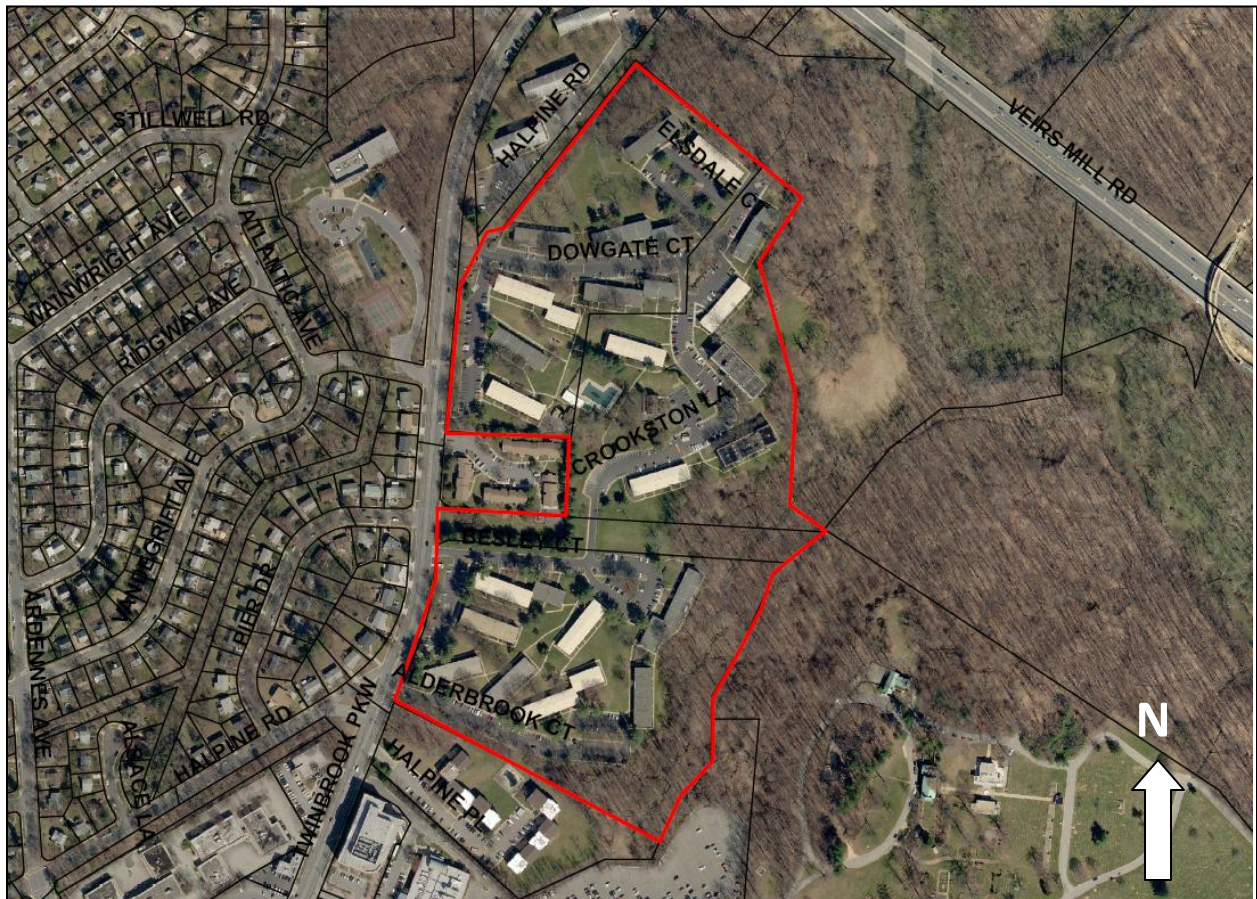
Site Aerial View
