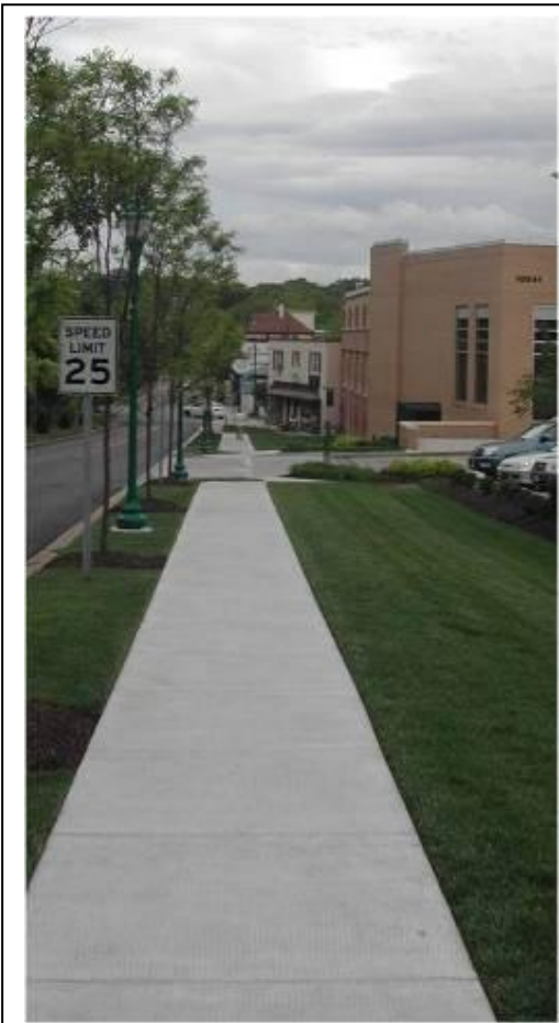
Existing Condition: Lack of building facades with display windows or entrances along this sidewalk on the Safeway property creates a dead zone.
