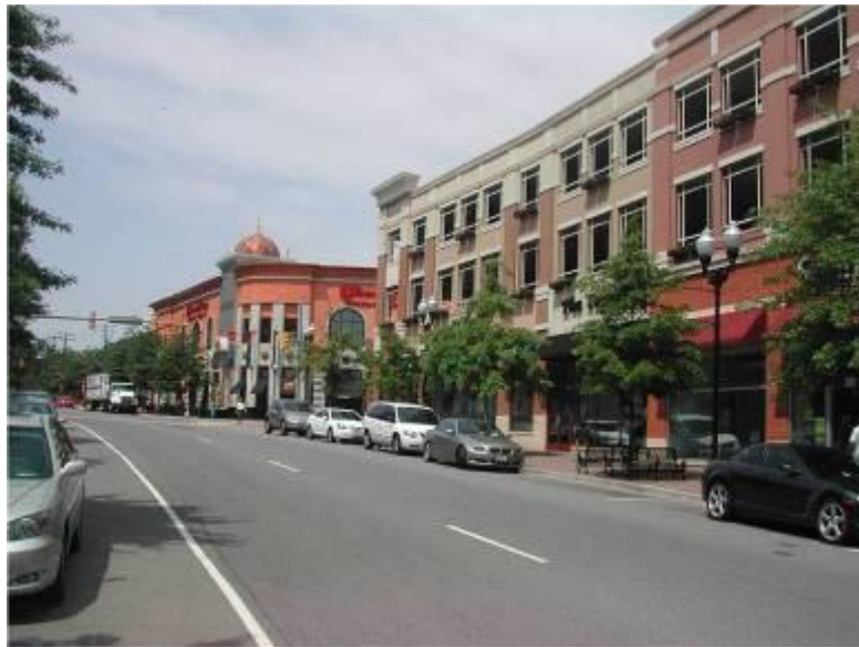
The punched window openings and planters create a traditional façade for this parking garage.
