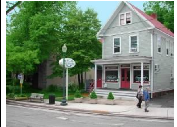
Building reuse at 10412 Montgomery Avenue.
