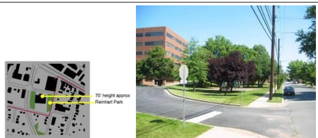
Existing Condition: Reinhart Park serves as a buffer between BCTGM Union building and structures along Armory Avenue.
