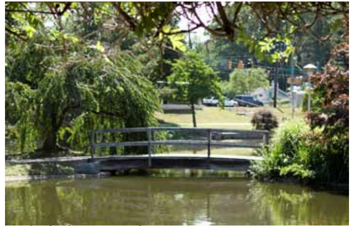
Existing bridge over pond
