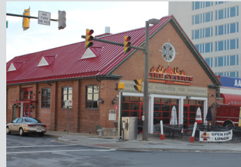
Adaptive Reuse: From a fire station to a restaurant
