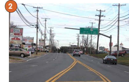
2 Lack of sidewalks
