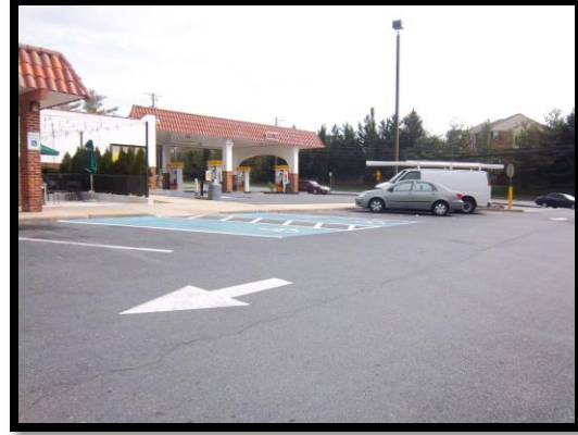
Figure 4: Shared drive-aisle southeast towards Bel Pre Rd
