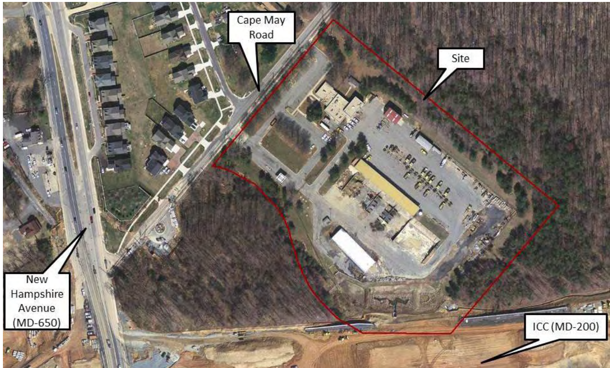
Figure 1: 2010 Aerial Photograph of Project Site and Vicinity
