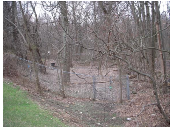
Figure 3: PB-33 SWM Facility retrofit
