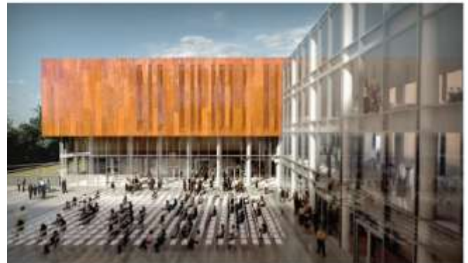
The south face viewed from Erskine.
