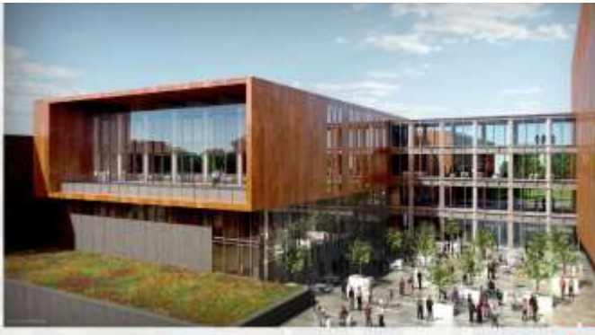
The west face, overlooking the Potomac. The Centrum is on the left with a glass connection to Erskine.
