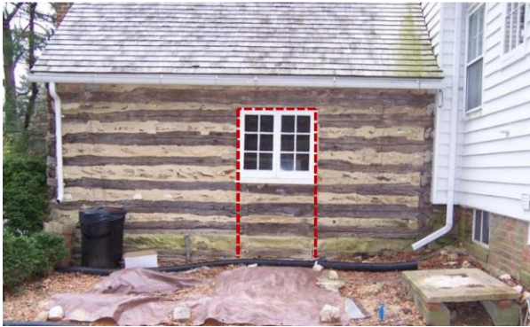
Figure 12: Log Kitchen, Visitor Exit
