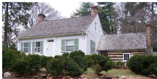
Figure 4: Riley/Bolten Historic House w/attached Log Kitchen
