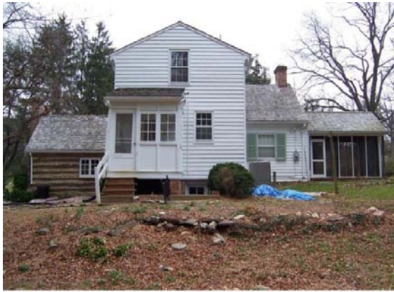
Figure 9: Riley/Bolten House - Rear Elevation
