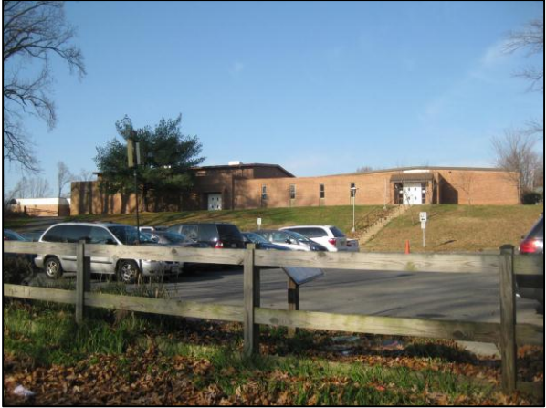
Parking area at Blaine Drive
