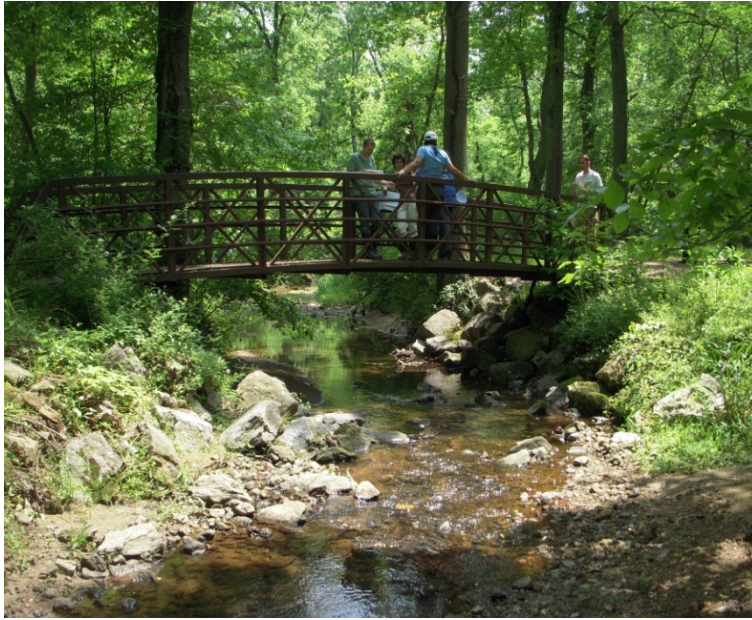
Existing pedestrian footbridge over Hollywood Branch
