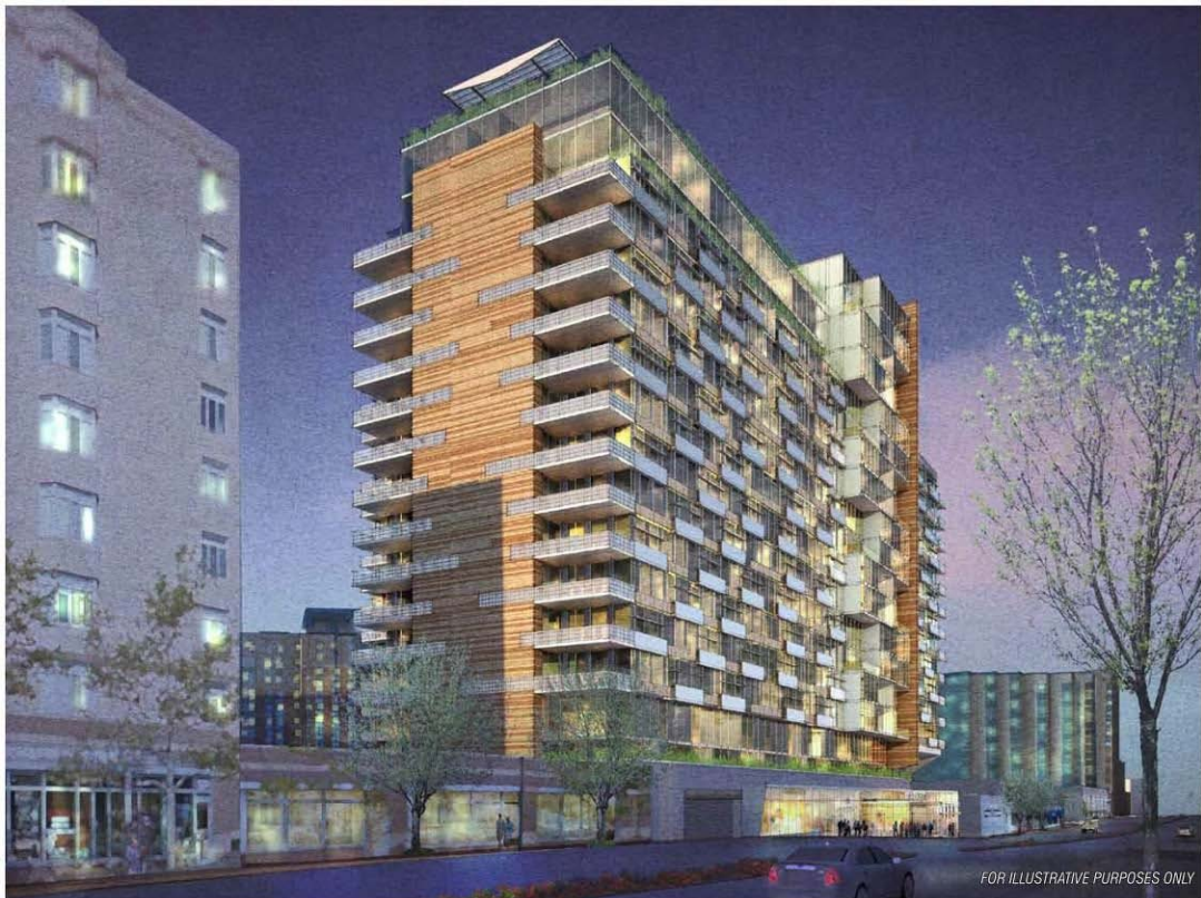
Wisconsin Avenue, looking north
