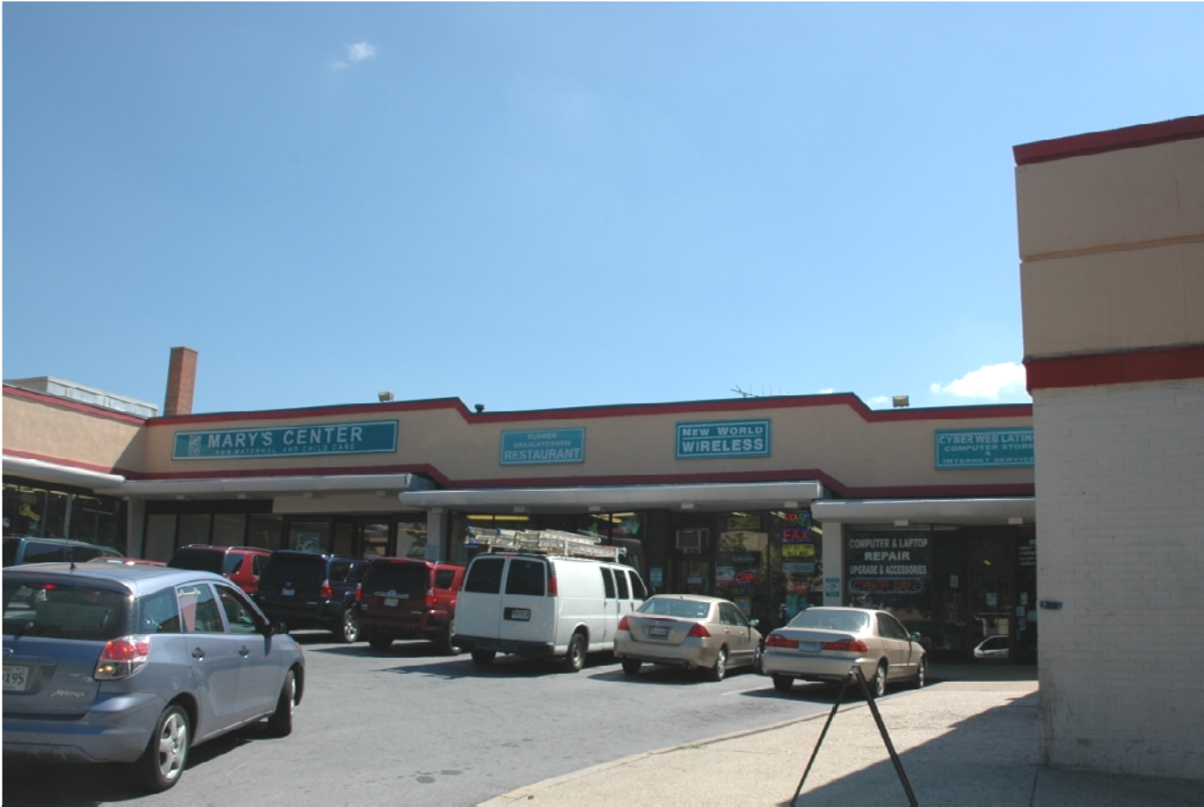
Arcaded shops with automobile forecourt parking. (Clare Lise Kelly, M-NCPPC, 6-2010)
