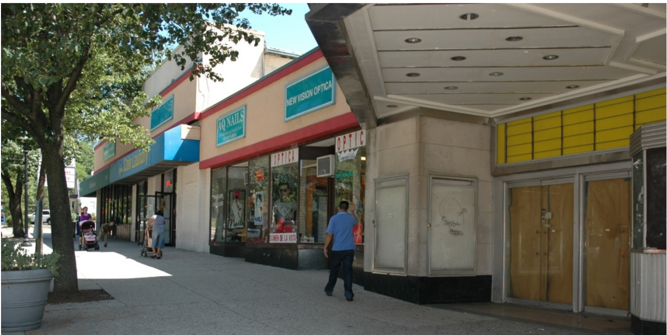
View north, from left to right: Giant Food Store, lobby shops, and theater entrance. (Clare Lise Kelly, M-NCPPC, 6-2010)
