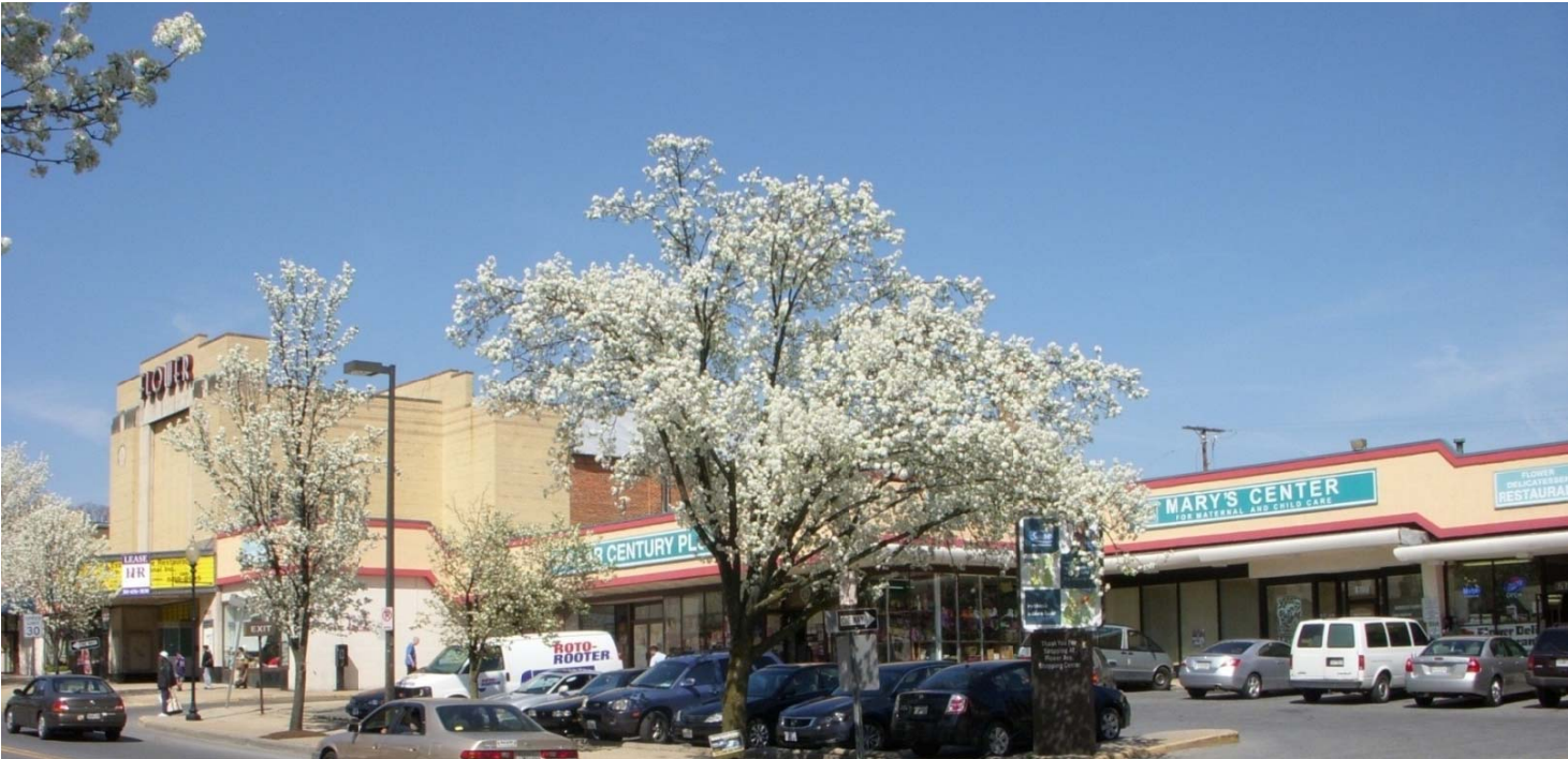
View from the southwest, from left to right: theater, barber shop, Woolworth’s, arcade. (Lisa Mroszczyk, M-NCPPC, 4-2010)
