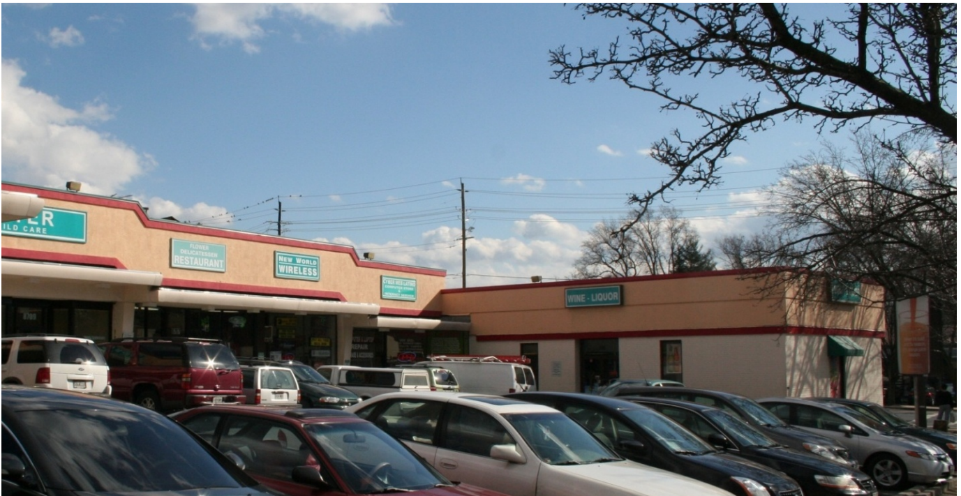
Storefronts in arcade at left, with north façade of former Whelan Drugstore, right, now a County Liquor Store. The walls have been sheathed in brick, though the entrance has been retained and metal cornice remains in place. (Clare Lise Kelly, M-NCPPC, 6-2010)
