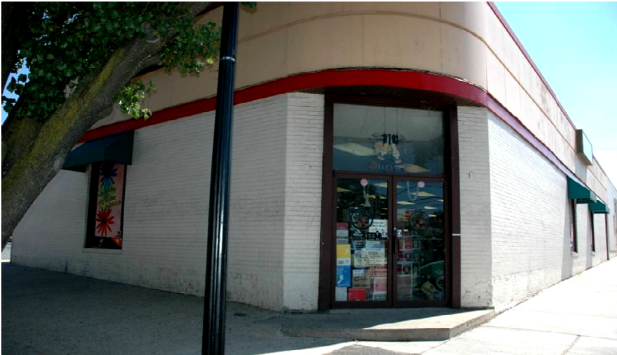
The original walls of the Whelan Drug Store building were replaced with brick facing and individual window units. Original features that remain include the curved metal cornice and the canted entrance that faces the corner of Piney Branch and Flower. (Clare Lise Kelly, M-NCPPC, 6-2010)
