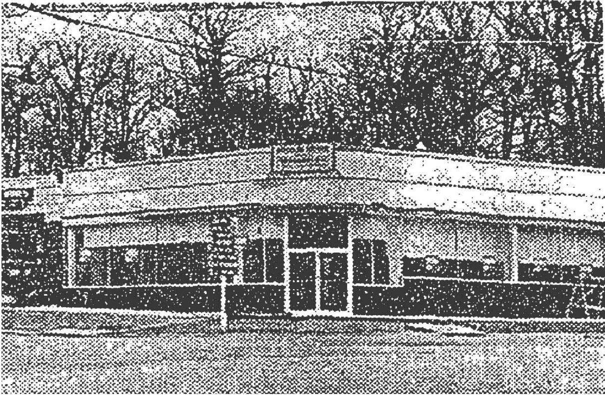
This detail of a 1950 photograph shows the Whelan Drug Store building with its wide metal cornice, canted corner entrance, and continuous windows. ( The Washington Post , January 15, 1950)
