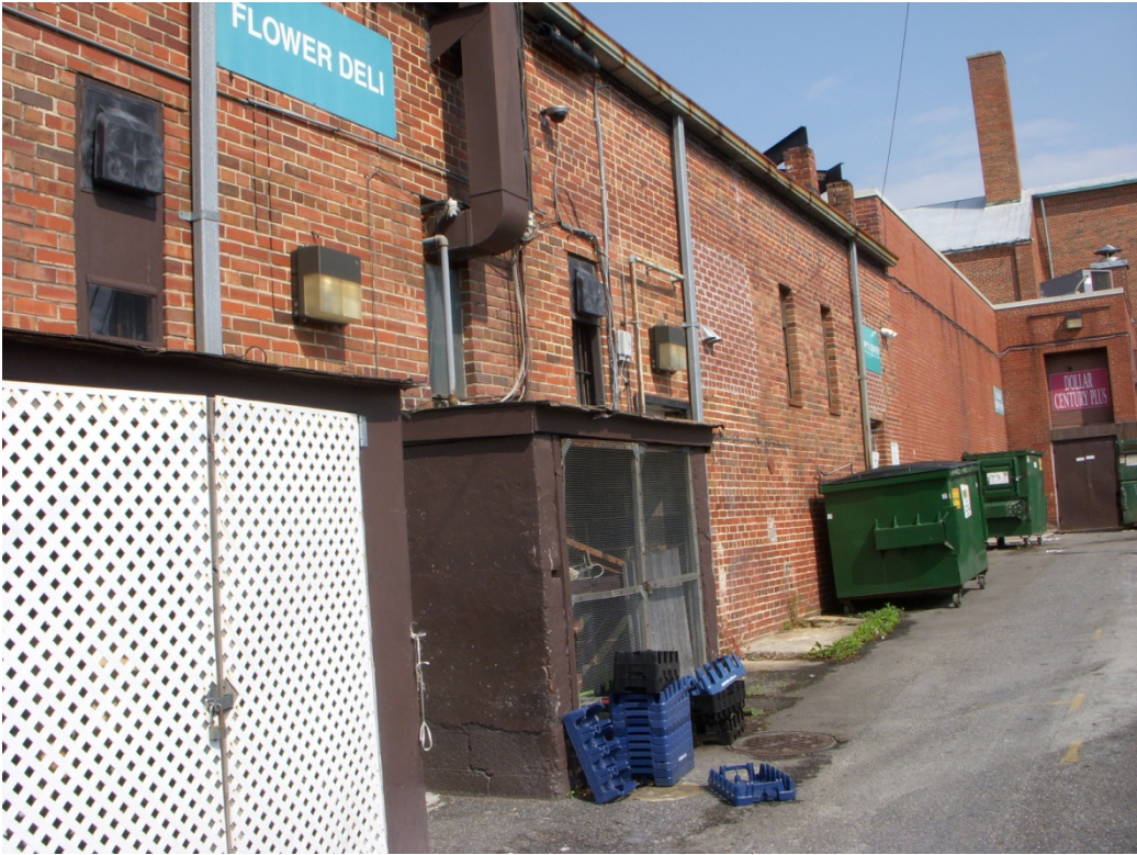
View north of east façade, with 8707 in foreground and theater in background, showing rear alley at right. (Lisa Mroszczyk, M-NCPPC, 4-2010)
