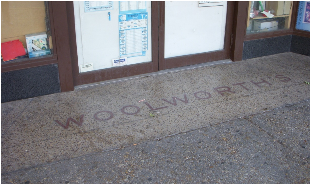
Woolworth's name is spelled out in the Terrazzo Floor of both entrances, west façade. (Lisa Mroszczyk, M-NCPPC, 5-2010)
